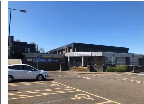
Exterior of building
