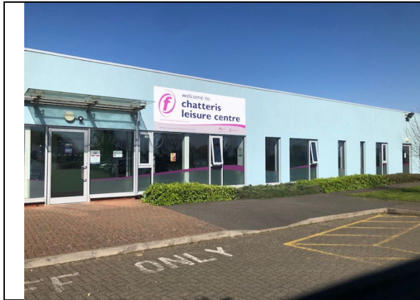
Exterior of building
