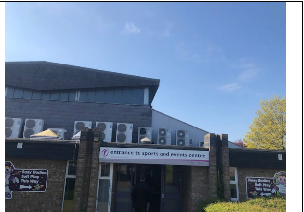
Exterior of dry side building
